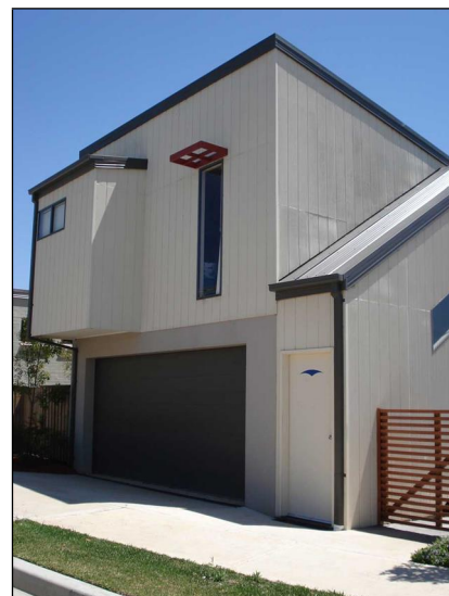
Figure 3 – Example of an Auxiliary Unit above a garage
