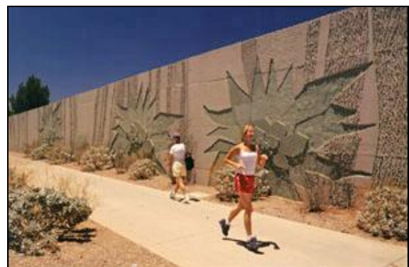
Figure 6.1 - High Quality Acoustic Barrier (Source: Dan Coogan - Pima Freeway 3, Scottsdale)
