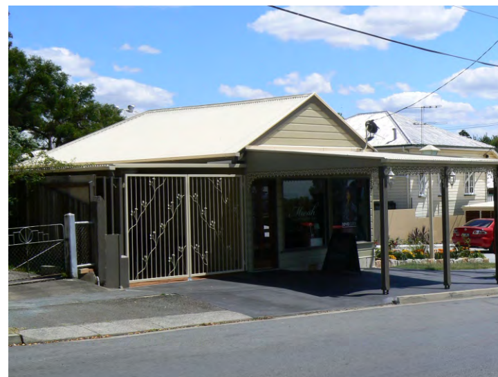
Presented to Brian Douglas for restoration of historic shops, 9 Blackstone Road, Eastern Heights.
