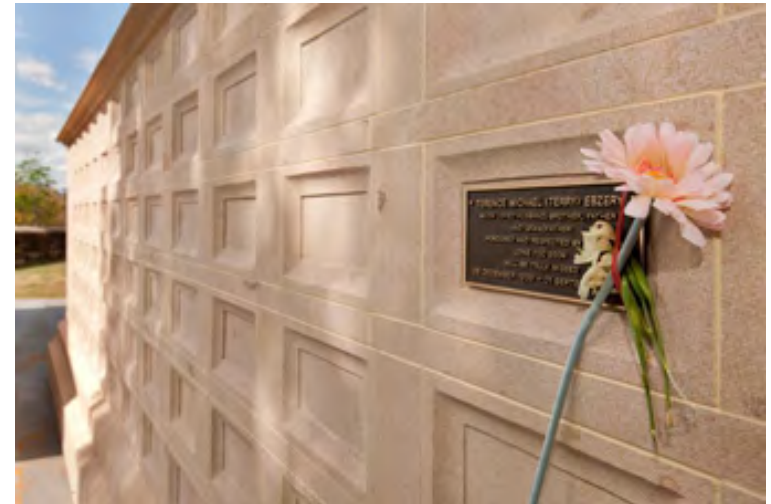
A Gold Award was presented to Thurlow Stonemasonry and JM Pearce Architects for 'St Mary's Columbarium'.
