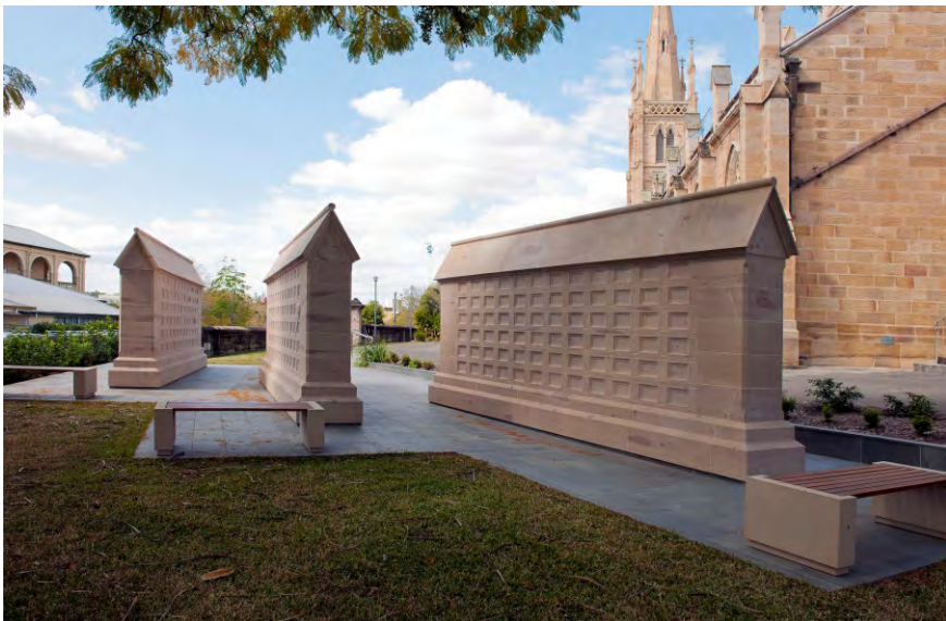
The Overall Heritage Award for Excellence was awarded to Thurlow Stonemasonry and JM Pearce Architects for St Mary's Columbarium.
